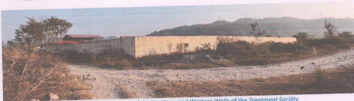
Figure 2: The intersection of the Northern and Western Walls of the Treatment Facility
