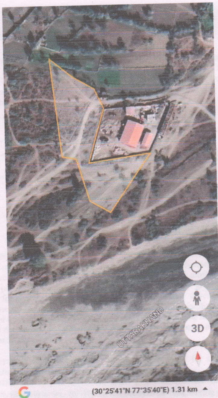
Figure 4: Google Earth Image of the Waste Treatment Facility and the adjoining polygon of proposed Miyawaki plantation
