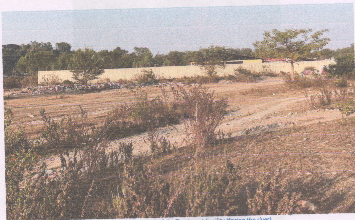
Figure 3: Southern Wall of the Treatment Facility (facing the river)
