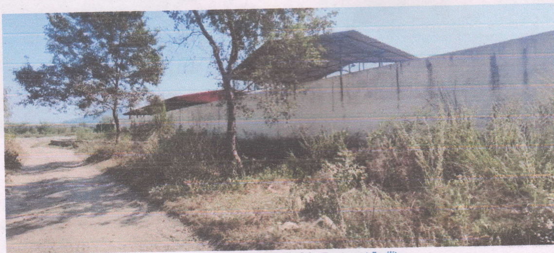
Figure 1: The Northern Wall of the Treatment Facility
